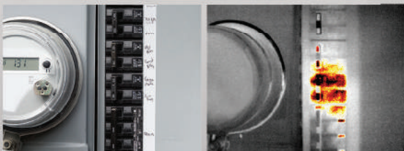
OVERLOADED CIRCUITS
